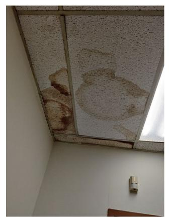
Figures 12a and 12b: Discolored ceiling tiles from leaky pipes.
