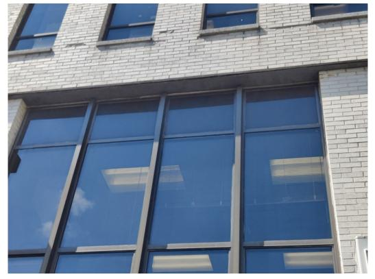
Figure 18: Area where the floor plate on the third floor is separating from the wall.
