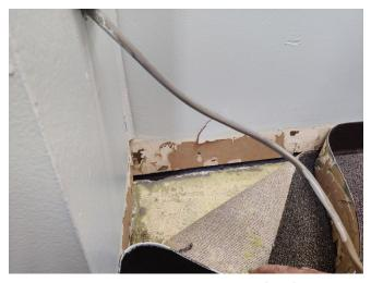
Figure 14: Area where interior wall is separating from floor plate.
